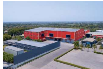
Quartz Sink Manufacturing Facility
